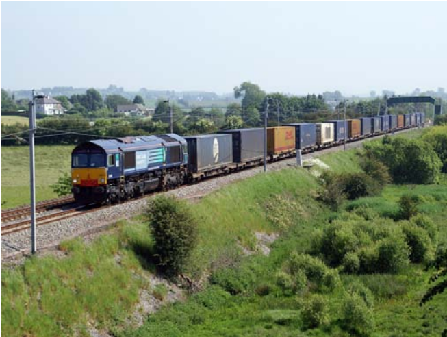
Direct Rail Services container service
